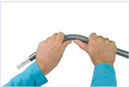
Bending with an external bending spring
