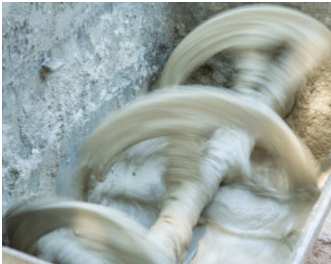
Mix Mapestone PFS 2 Flex only with water using a mixing drill or concrete mixer
