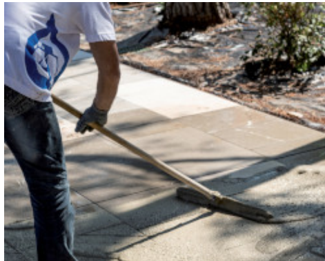
Application of Mapestone PFS2 Flex on slab paving previously wetted with water
