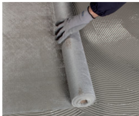
Placing Mapetex Sel N on the first coat of Mapelastic Turbo while till wet
