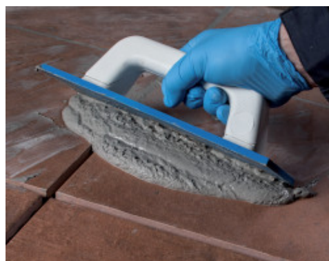
Placing Mapetex Sel N on the first coat of Mapelastic Turbo while till wet
