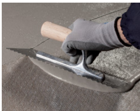
Application of the second coat of Mapelastic Turbo over the first coat reinforced with Mapetex Sel N
