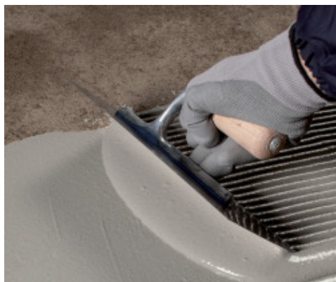
Application of the first coat of Mapelastic Turbo
