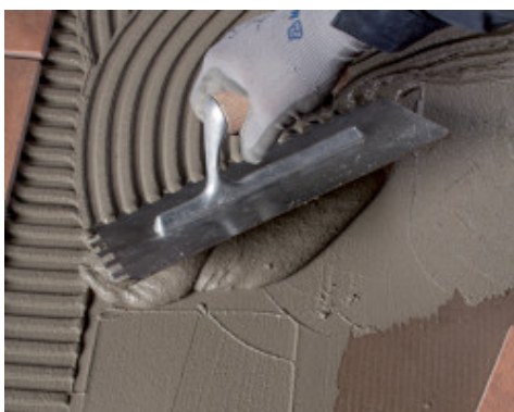
Placing Mapenet 150 on the first coat of Mapelastic Turbo while till wet
