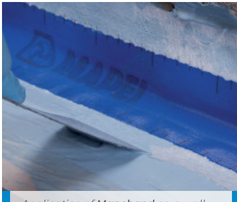
Application of Mapeband on a wall-floor fillet joint with Mapelastick AquaDefense
