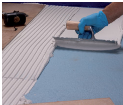
Bonding tiles on Mapelastic AquaDefense
