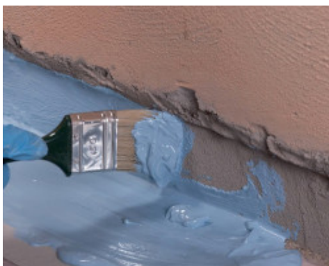
Application of Mapelastic AquaDefense by brush between floor and wall before applying Mapeband
