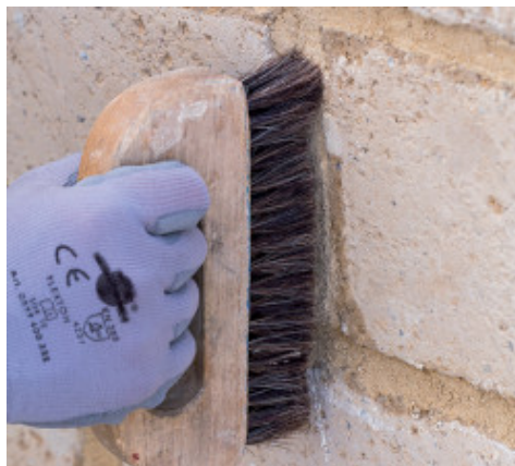
Finishing the mortar joints
