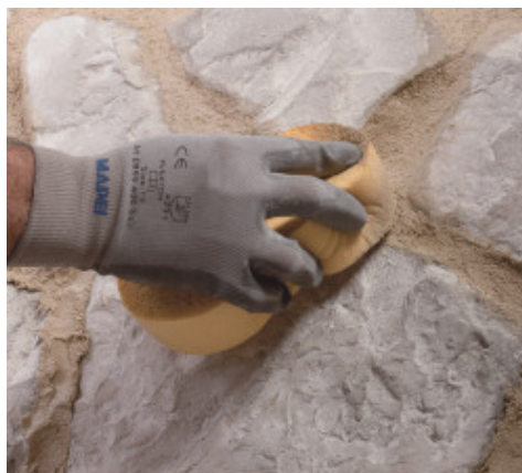
Finishing the surface with a sponge
