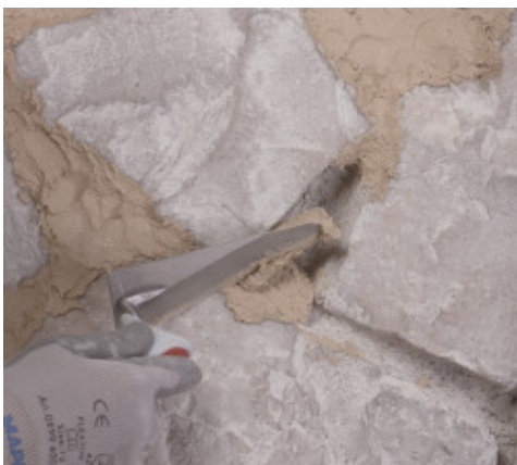
Pointing the joint in a stone wall
