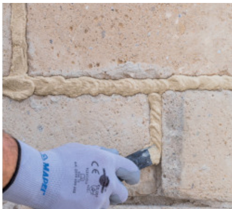
Removing the excess mortar
