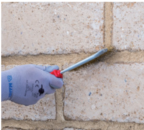
Brushing the mortar joints
