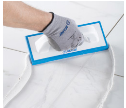
Easy-to-apply epoxy grout
