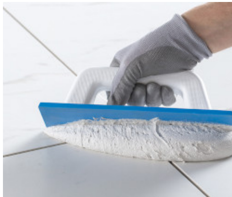
Spread Kerapoxy Easy Design with Mapei trowel
