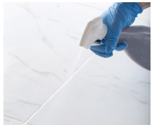
Possible final cleaning with UltraCare Kerapoxy Cleaner
