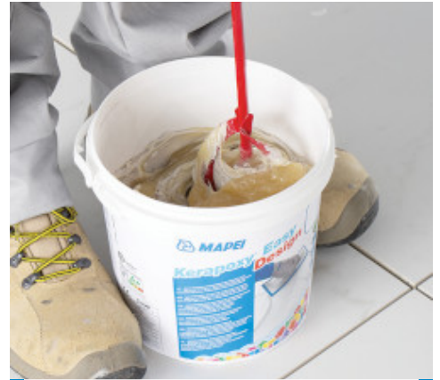
Mix the components (A+B)
