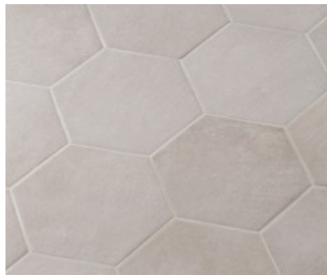
Floor grouted with Keracolor FF
