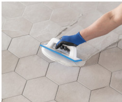
Application of Keracolor FF with MAPEI float
