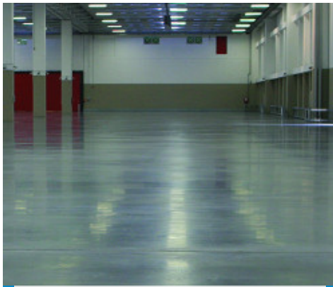
Example of industrial flooring admixed with Mapefibre NS12
