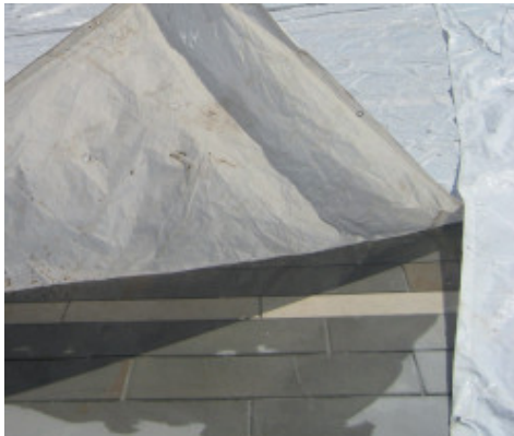
Example of pavement protection
