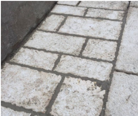
Flagstones grouted with Mapestone PFS 2 Visco
