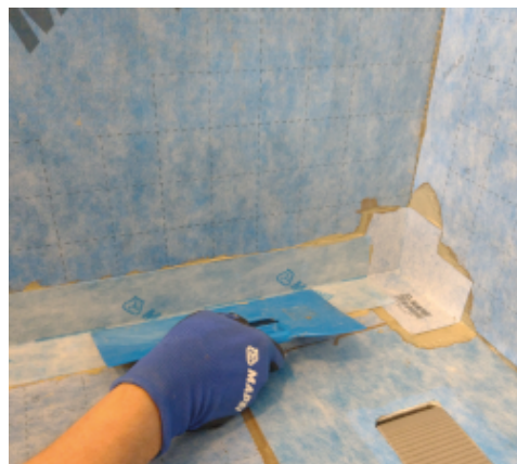
Application of Mapeguard ST
