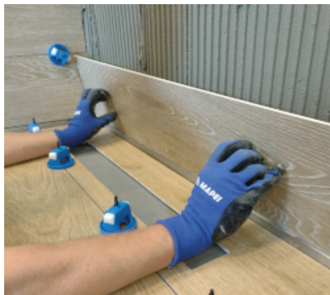
Installation of tiles
