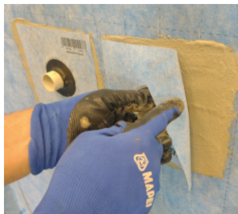
Application of Mapeguard PC
