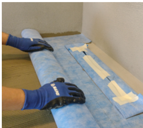
Application of Mapeguard WP 200
