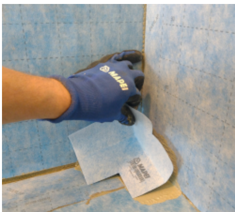
Application of Mapeguard IC
