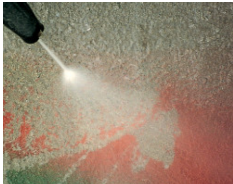
Using high-pressure cleaner on concrete treated with WallGard Graffiti Barrier
