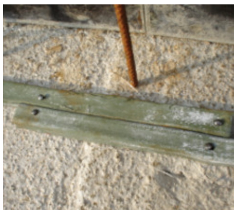
Overlapping the ends of Idrostop B25
