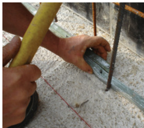
Overlapping the ends of Idrostop B25
