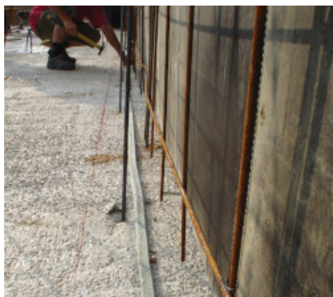
Laying Idrostop B25
