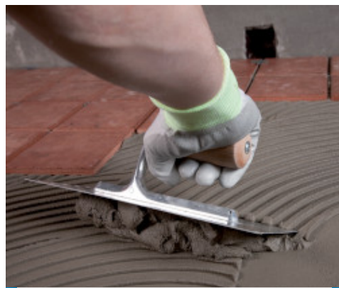
Application of Granirapid on terrace waterproofed with Mapelastic
