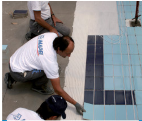
Application of ceramic coating on Mapelastic
