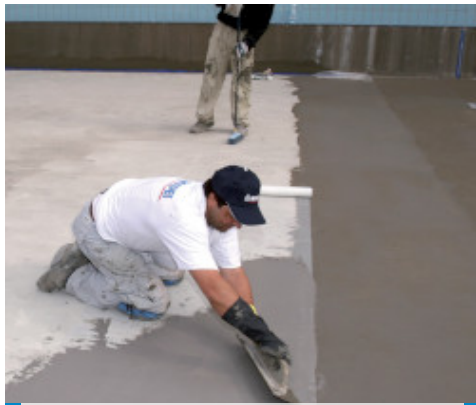
Waterproofing a swimming pool with Mapelastic
