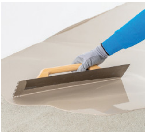
Nanošenje mase Ultraplan Contract
