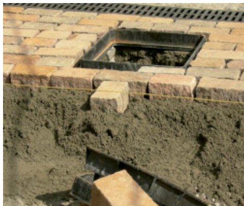
Mapestone TFB 60 mixed to a "no-slump" consistency
