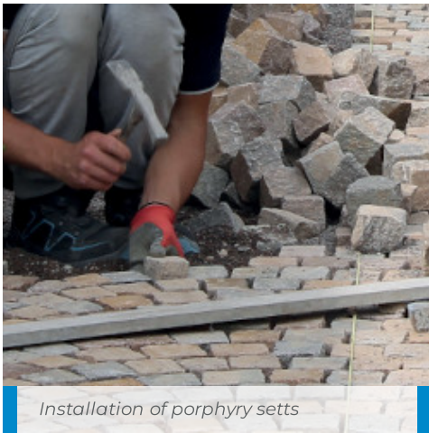
Close-up of setts installation
