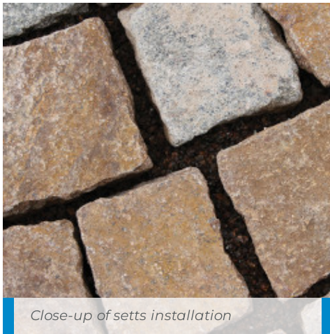
Filling the joints with gravel
