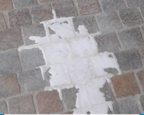
Staining cleaning on porphyry cubes: apply Mapestone Scraper for 5-10 minutes
