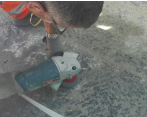
Mechanical abrasion, before applying Mapestone Scraper in case of exceeding residues
